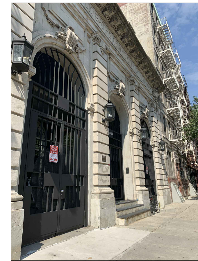
D FACADE, PHOTO FROM SIDEWALK SCALE: N/A
