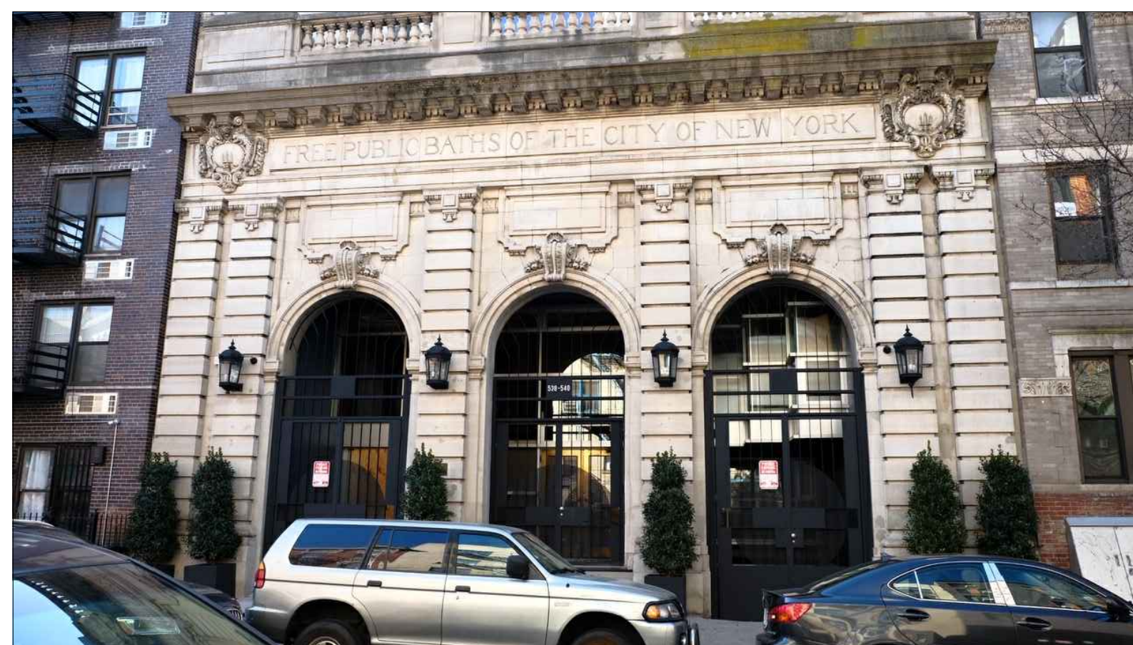
B FACADE, PHOTO FROM STREET SCALE: N/A
